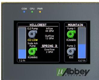
At both Mountain & Hillcrest Reservoirs there are local touch screen displays connected to the Swampfox RTU. These display Reservoir levels, pump status and flows in the system.
